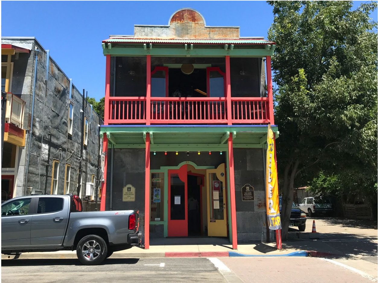
A modern tap room occupies an 1870s former opium den in Isleton. (Stacy Hayden/Delta Protection Commission)
